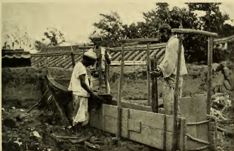
BRICK LAYING EXTRAORDINARY
